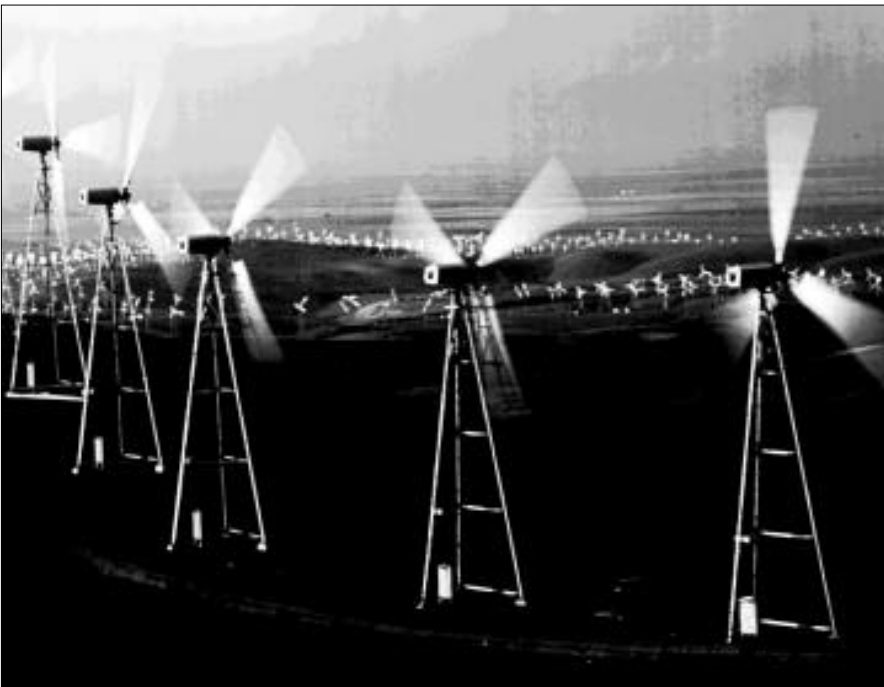
This wind farm uses many wind turbines to produce electricity.
