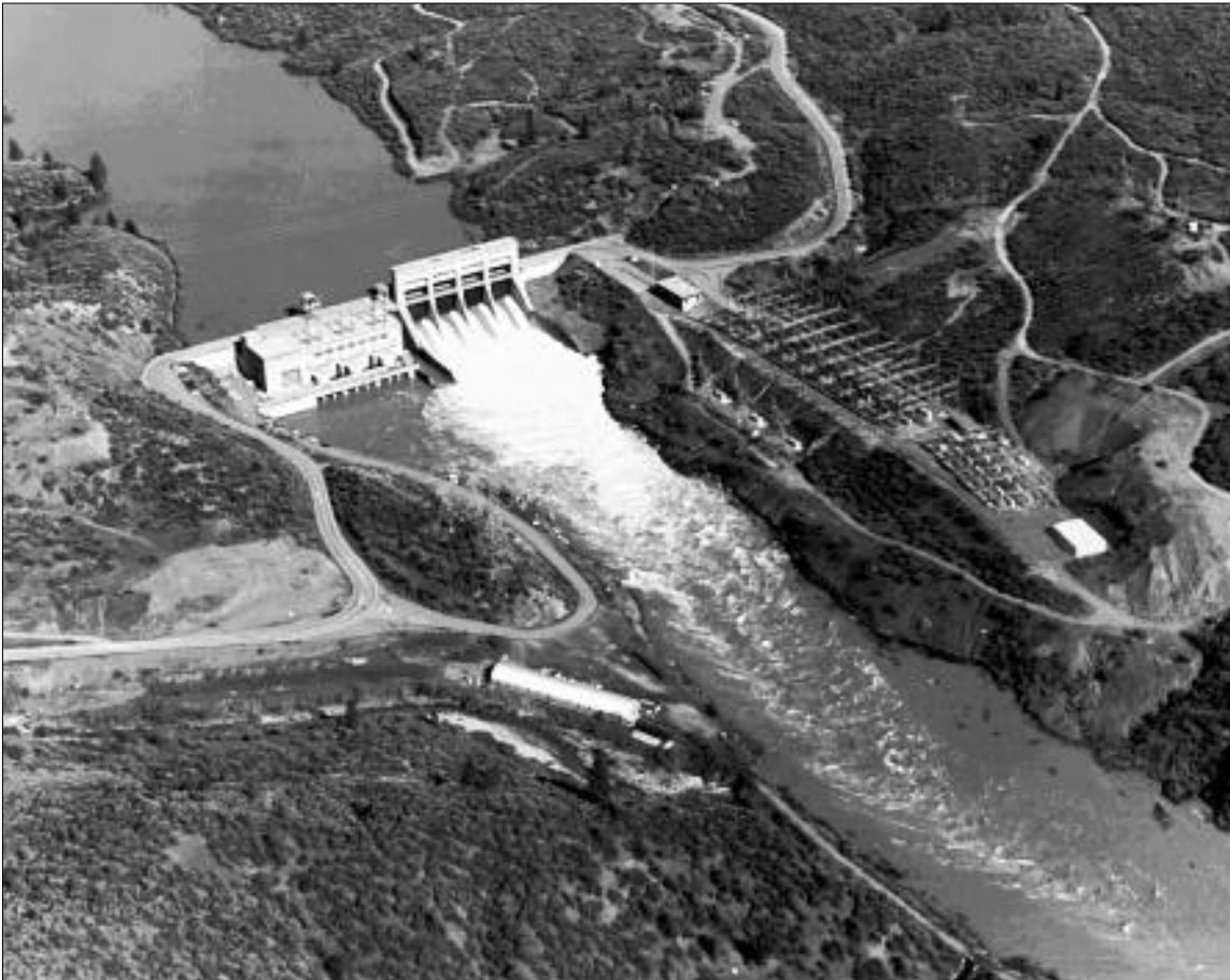
This hydropower plant is located at the Keswick Dam on the Sacramento River north of Redding, California.
