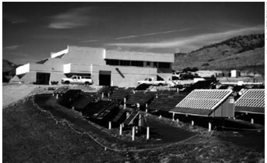
At NREL's Outdoor Test Facility, photovoltaic modules and systems made by various manufacturers and using various technologies are tested and monitored under actual weather conditions, as well as under controlled laboratory and accelerated weathering conditions.
