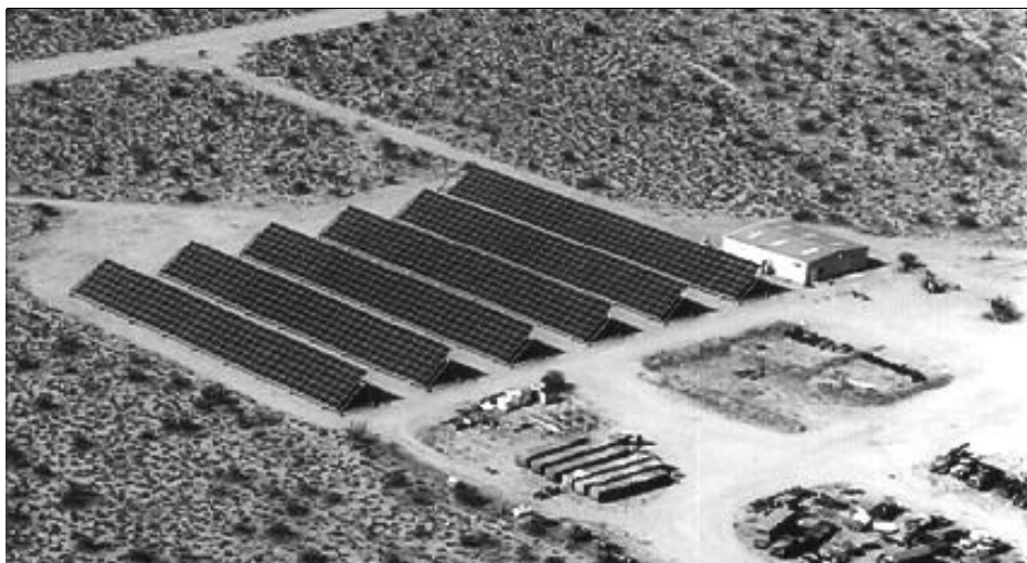
This 290-kilowatt PV hybrid system stemming from PV Program activities generates electricity for a military operation in China Lake, California.
