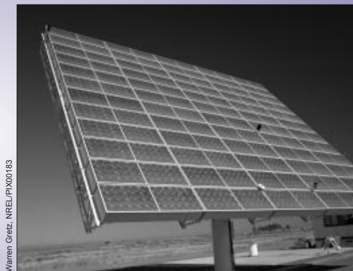
This PV concentrator tracking system is currently deployed at PVUSA in northern California.
