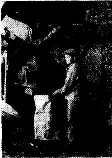
Figure 59. Packing Generator Gas Charcoal
