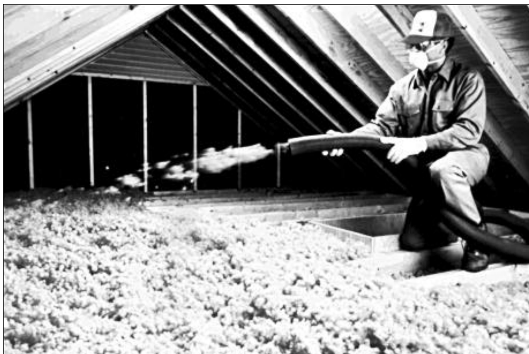
Loose-fill insulation is typically installed with special equipment that forces it through a hose at the proper density.
