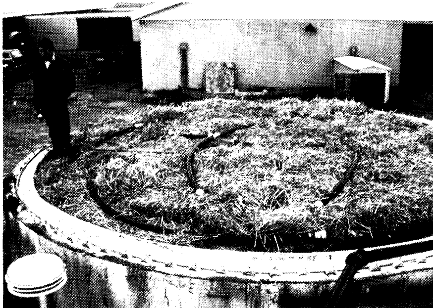
Figure 3-5. The 110-m 3 Dry Fermentation Shown Loaded with Straw Prior to Installation of the Cover. The distribution grid through which leachate was recycled for moisture and temperature control is visible
