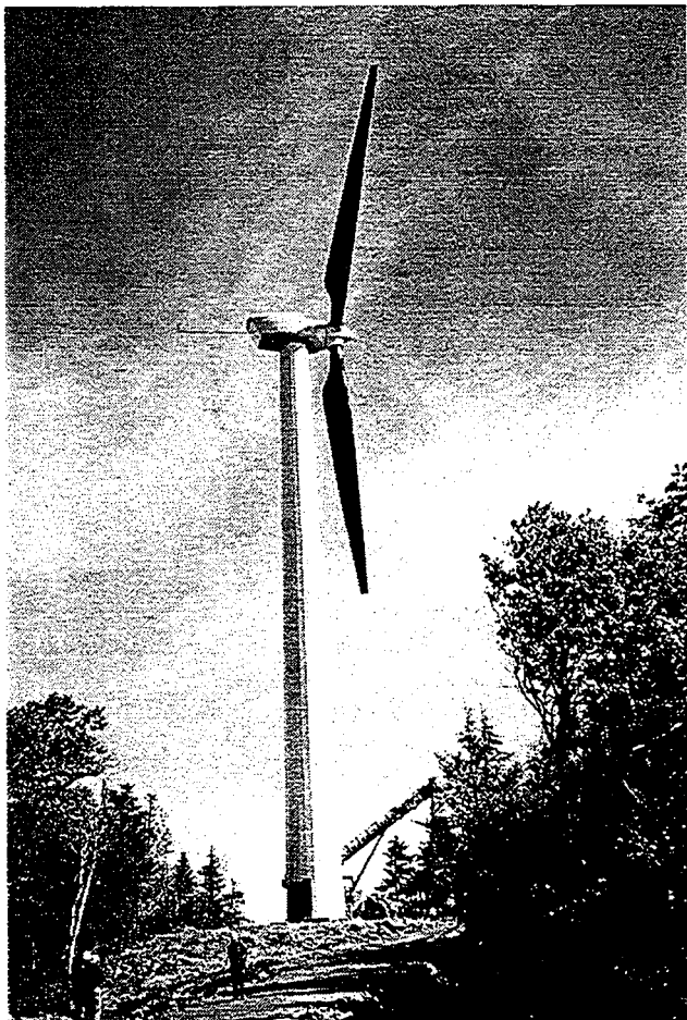
FIG. 2. A ZOND Z-40FS WIND TURBINE AT THE GREEN MOUNTAIN POWER WIND PLANT NEAR SEARSBURG, VERMONT. SPECIALLY COATED BLACK BLADES REDUCE ICING.
