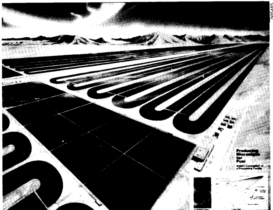
Figure 2-1. Artist's Conception of Microalgae Production Facility Located in the Southwest United States
