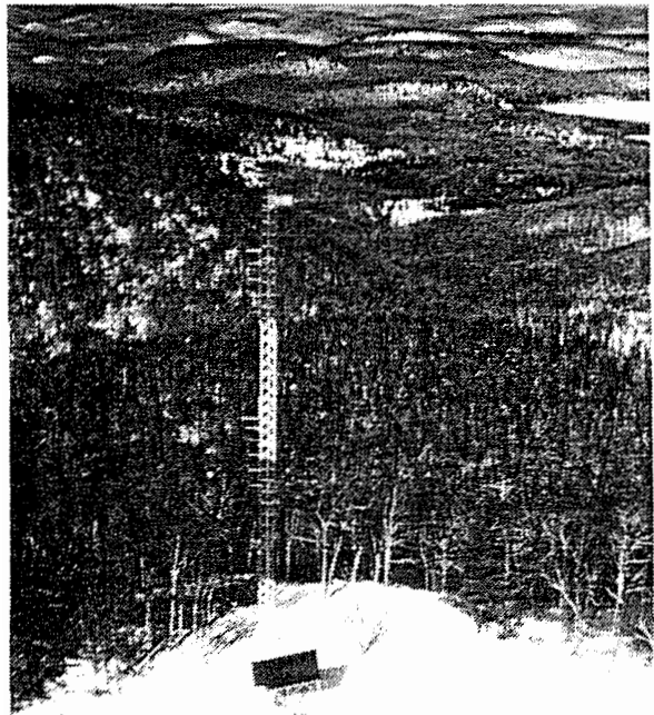
Fig. 9. Power for telecommunications and remote signals constitutes the largest market sector for PV power modules today. Photo shows radio communications in Northern Canada.
