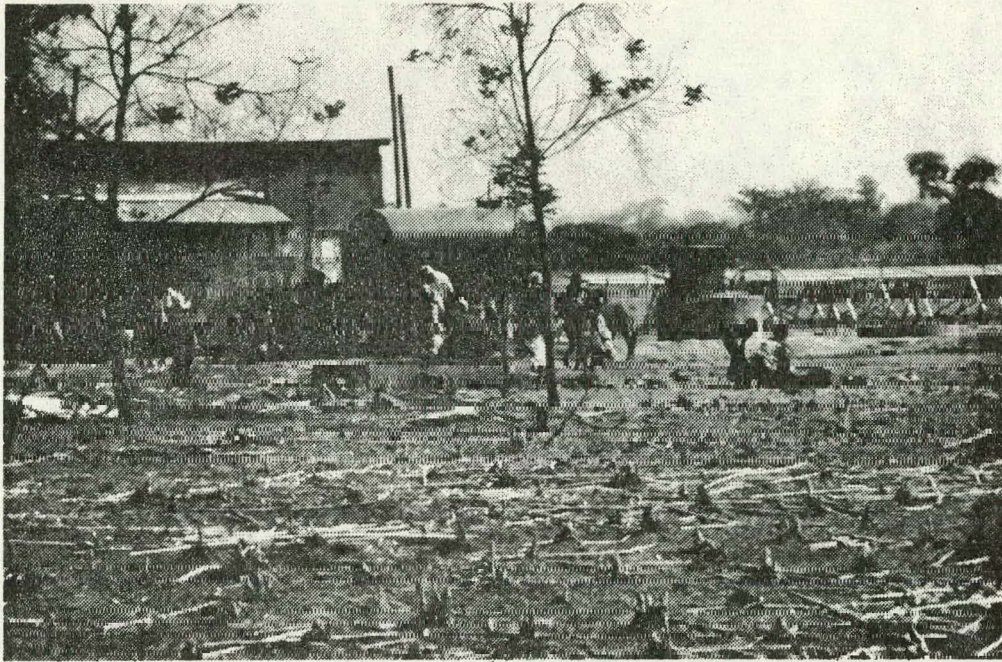
Figure 3-6. A view of the 1.8-kW p solar cell arrays (right center) in the village of Tangaye, Upper Volta, which power a water pump and a grain mill. The pump supplies the water dispensing tank (center). The grain mill, operated as a cooperative by the village, is located in the building behind the tank.
