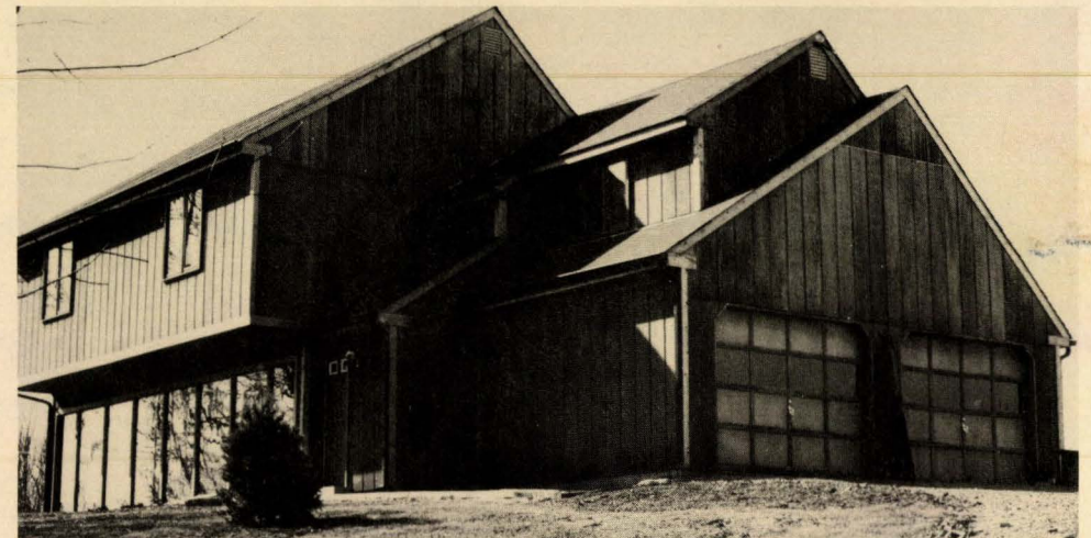
A thermal storage wall blends in well with the conventional design of this 1,800-square foot home in Glen Mills, Pennsylvania. The inner surface of the wall is painted to complement the decor of the living room behind it; several well-placed windows admit sunlight. Residents of the house paid a total of $200 for heating and hot water during the 1978-79 heating season. The builder estimates the house cost $3 to $4 more per square foot than a conventional house in the area, yet homeowners can save 60% in heating bills. Designer—Jim Kries, Sunburst; Photo—NSHCIC
