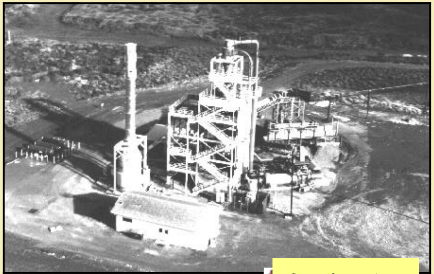
This gasification plant in Hawaii will initially process bagasse from the neighboring sugarcane refineries, but is designed to receive a wide variety of biomass.
